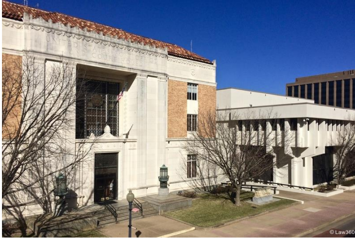
Buildings of the U.S. District Court for the Eastern District of Texas in Tyler, Texas. (Jess Krochtengel | Law360)
